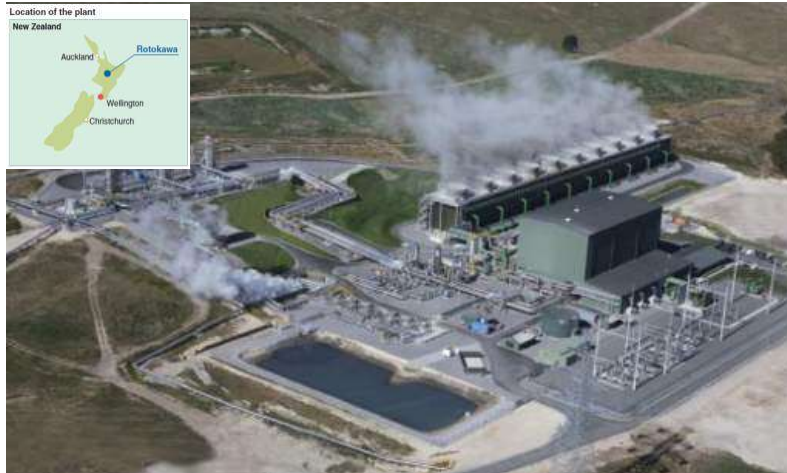
Nga Awa Purua Geothermal Power Station (The world's largest geothermal power station)
